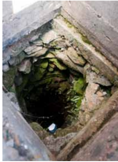
LEFT: The concrete frame was added to the stone well sometime in the early- to mid-20th century and originally supported a windlass used to draw up water. RIGHT: Roughly two miles from the well is the gravesite of Crockett's first wife, Polly.
